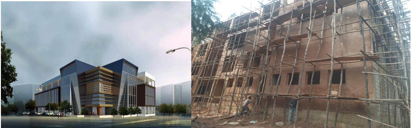
Figure: photo that shows status of construction G+3 office building
