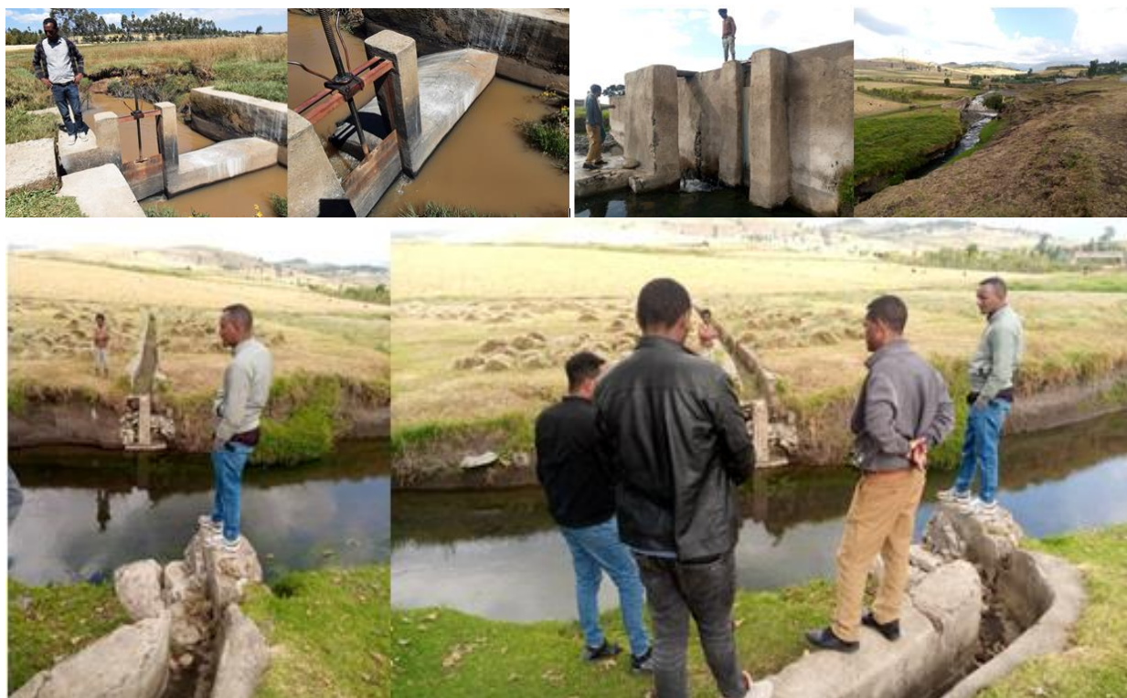
Figure 33. Shows during Assessment of schemes and diversion weirs
