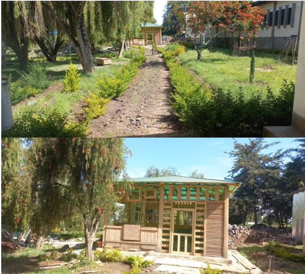
Partial view of recreational area under construction
