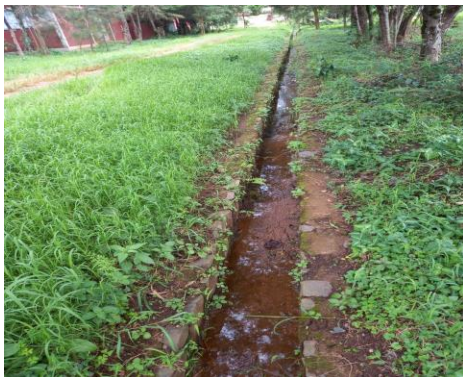
Cleared flood ditch
