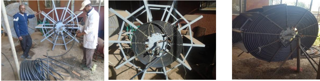
Fig 2: Shows fabrication processes
