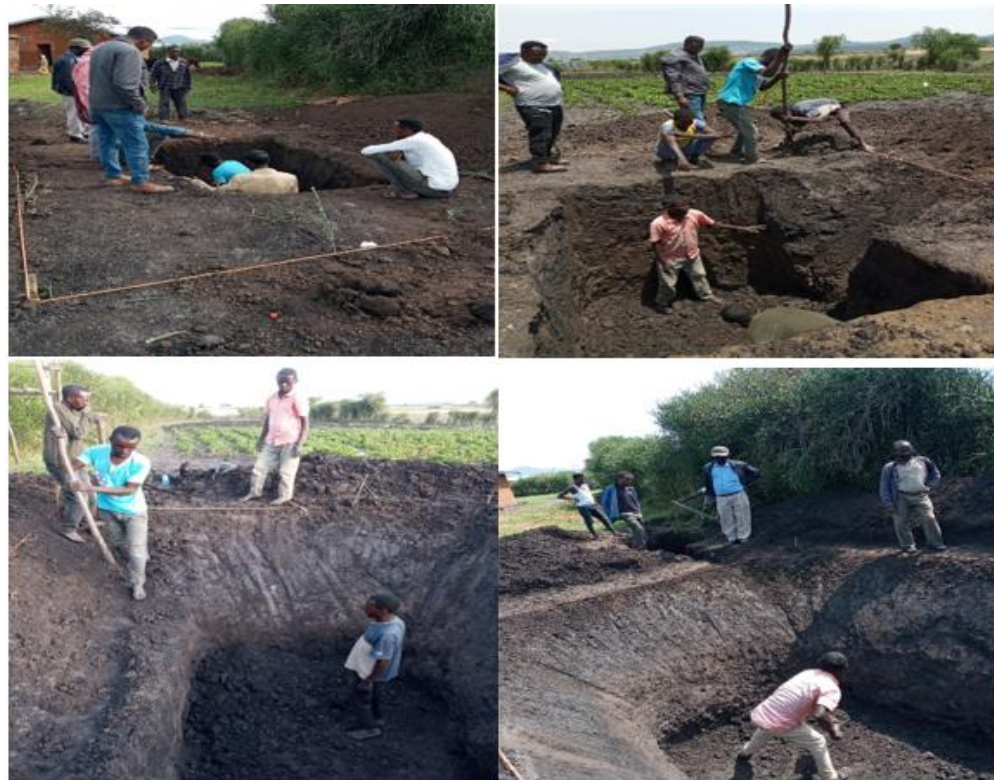
Figure 15: Constricting ponds for the surface runoff harvesting
