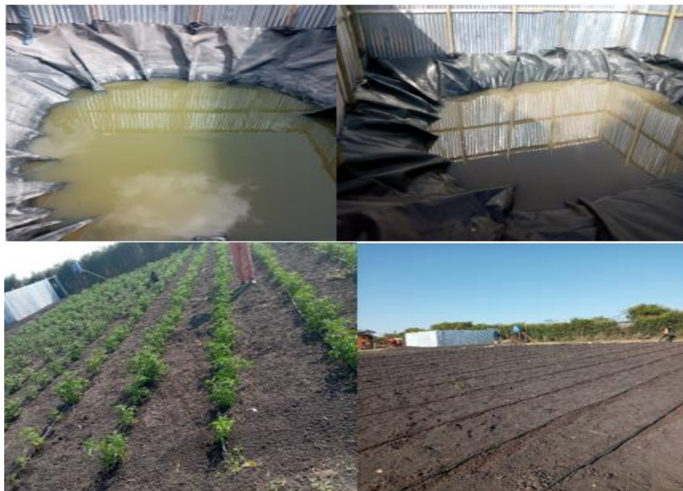
Figure 16: Harvested water used for Irrigation by Drip irrigation
